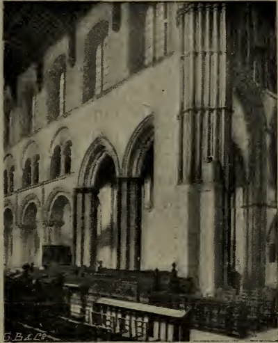
NAVE, NORTH SIDE.
